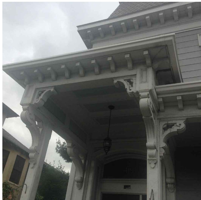
④ VIEW OF EXISTING FRONT PORCH ROOF
